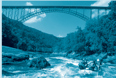
Rafters under New River Gorge Bridge.
