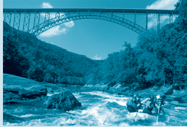
Rafters under New River Gorge Bridge.
